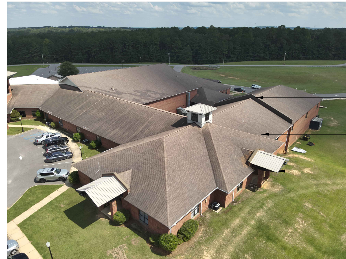
RIGHT FRONT CORNER
