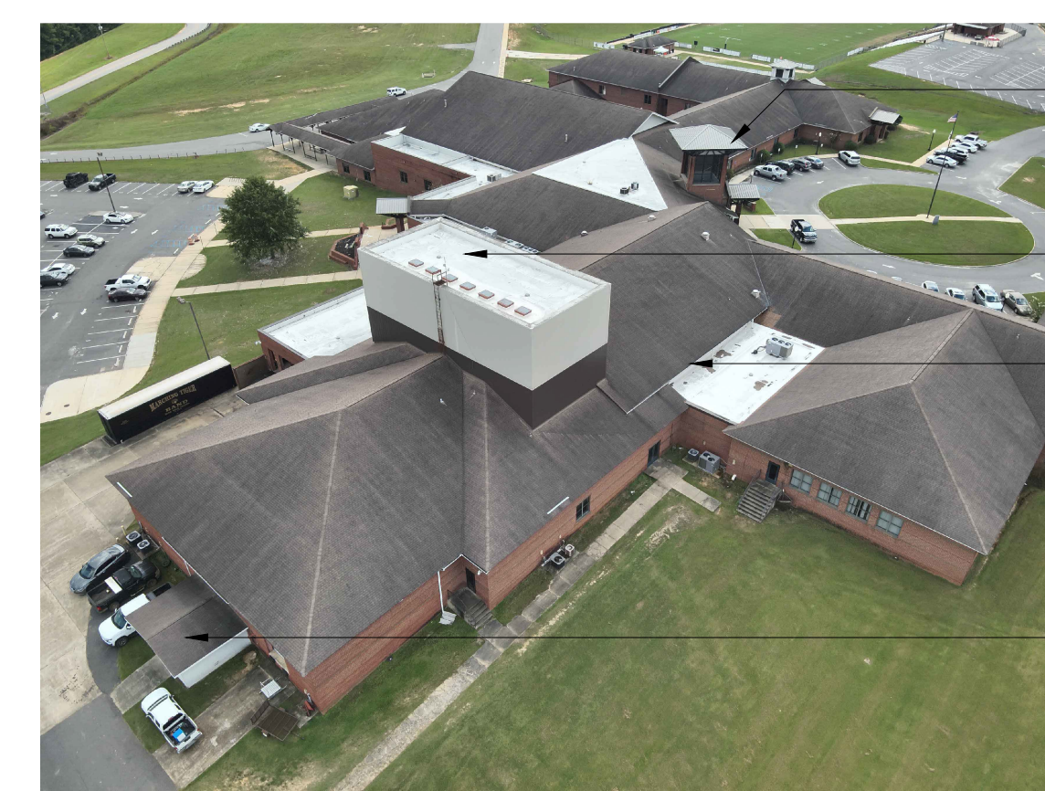
REAR CORNER VIEW
