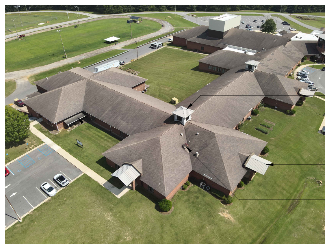
LEFT SIDE OF BUILDING
