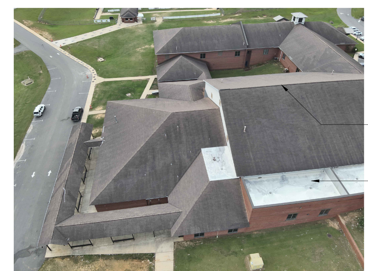
REAR CORNER VIEW
