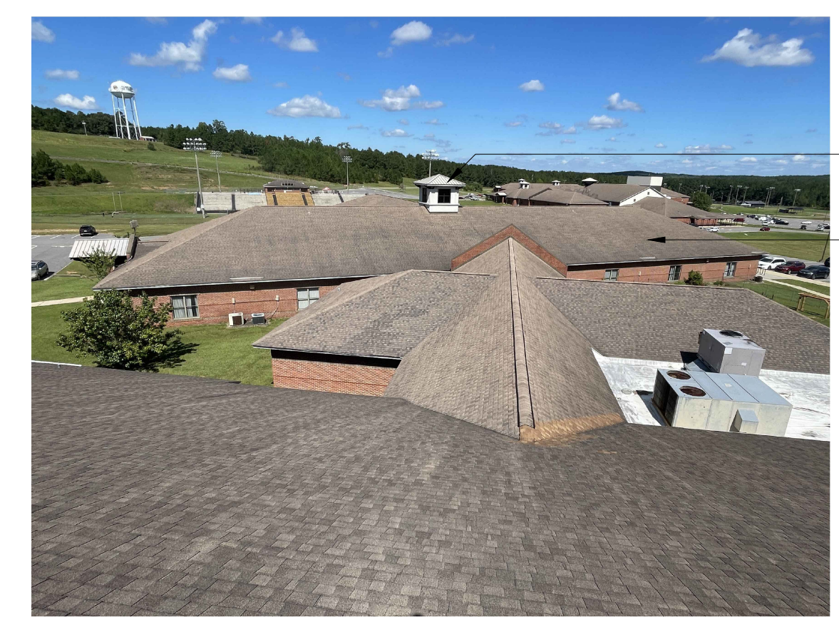
RIGHT SIDE VIEW (LOOKING OVER FLAT ROOF OF CENTER BUILDING)
