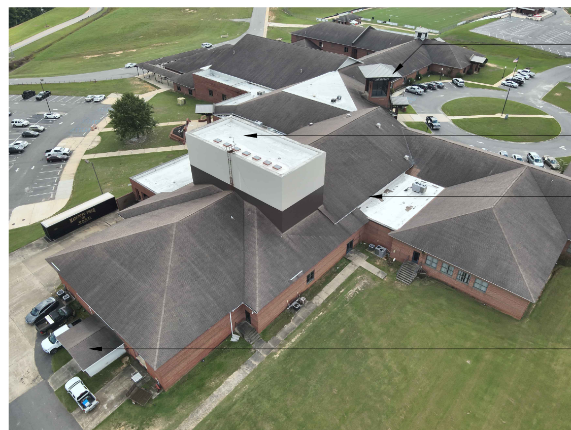
REAR CORNER VIEW
