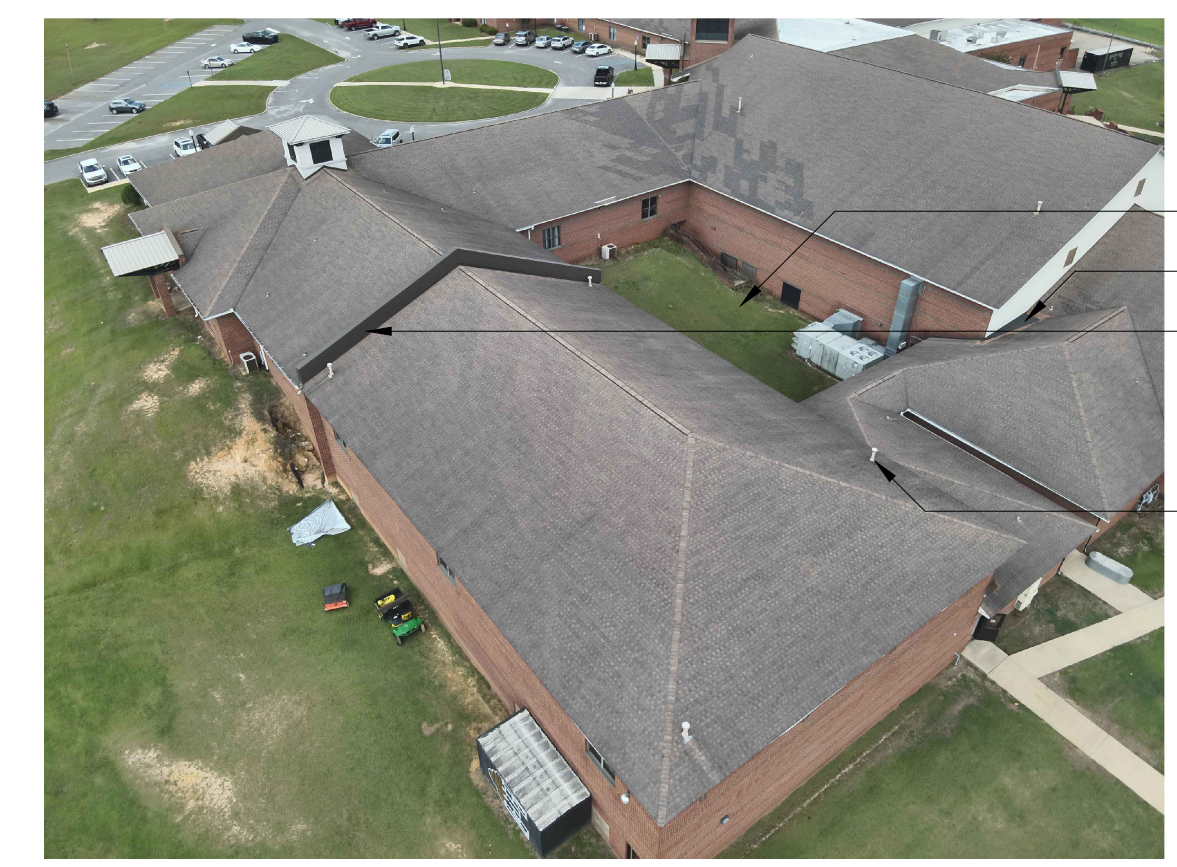
RIGHT REAR CORNER VIEW
