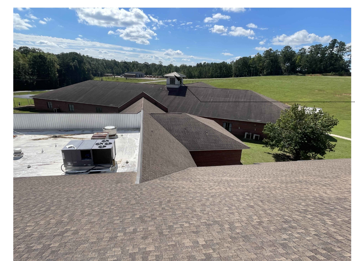
LEFT SIDE VIEW (LOOKING OVER FLAT ROOF OF CENTER BUILDING)
