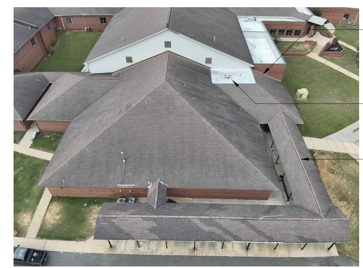
REAR RIGHT SIDE AT COVERED WALKWAY
