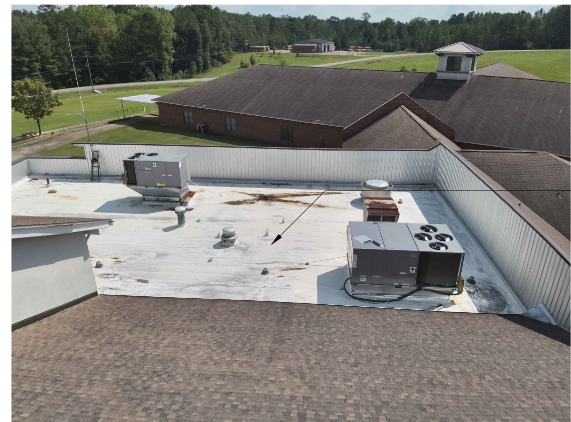
LOW SLOPED ROOF ON RIGHT SIDE OF BUILDING
