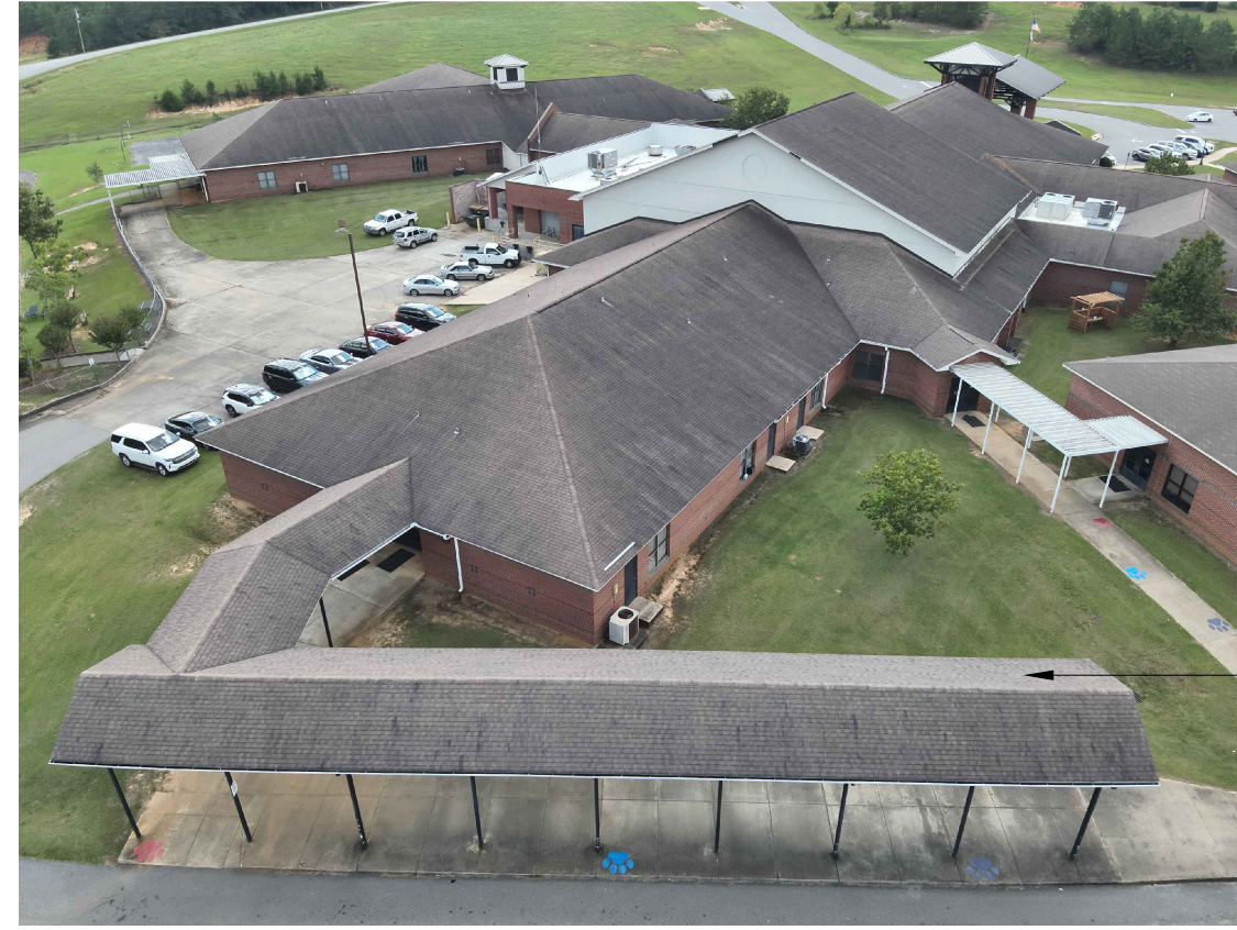
REAR COVERED WALKWAY
