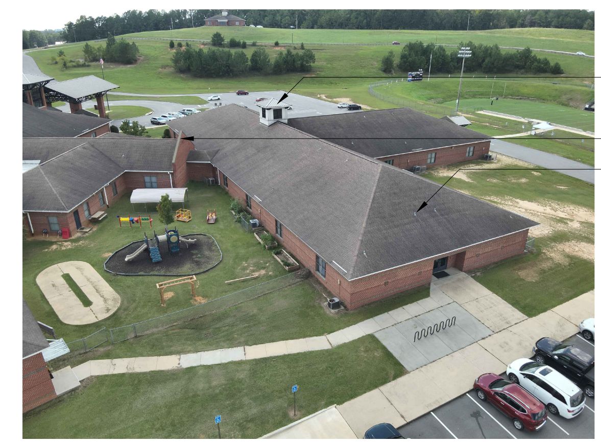
REAR CORNER VIEW
