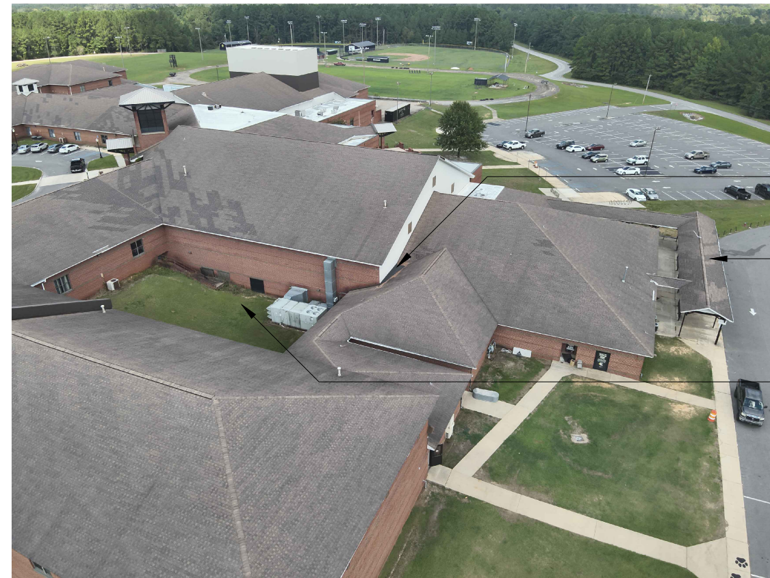
REAR RIGHT CORNER WITH COVERED WALKWAY
