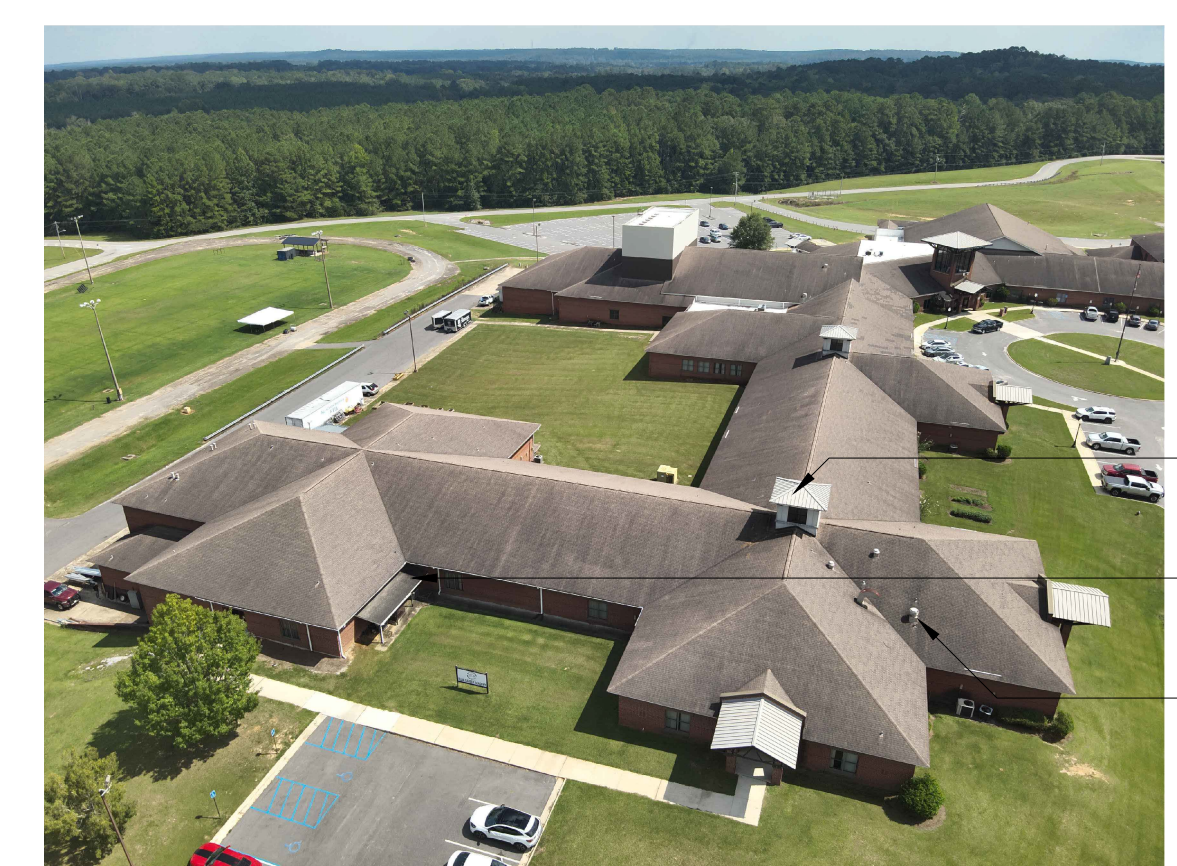
LEFT SIDE OF BUILDING
