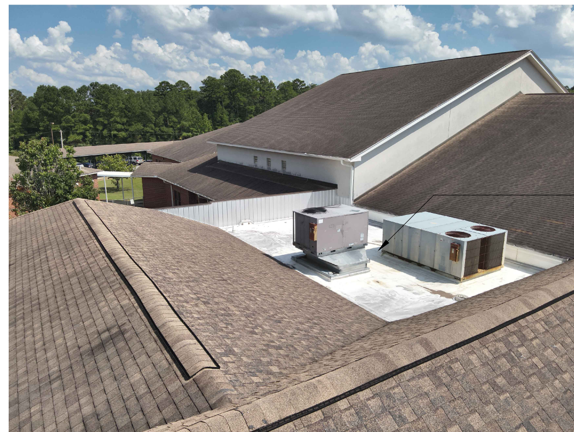
LOW SLOPED ROOF ON LEFT SIDE OF BUILDING
