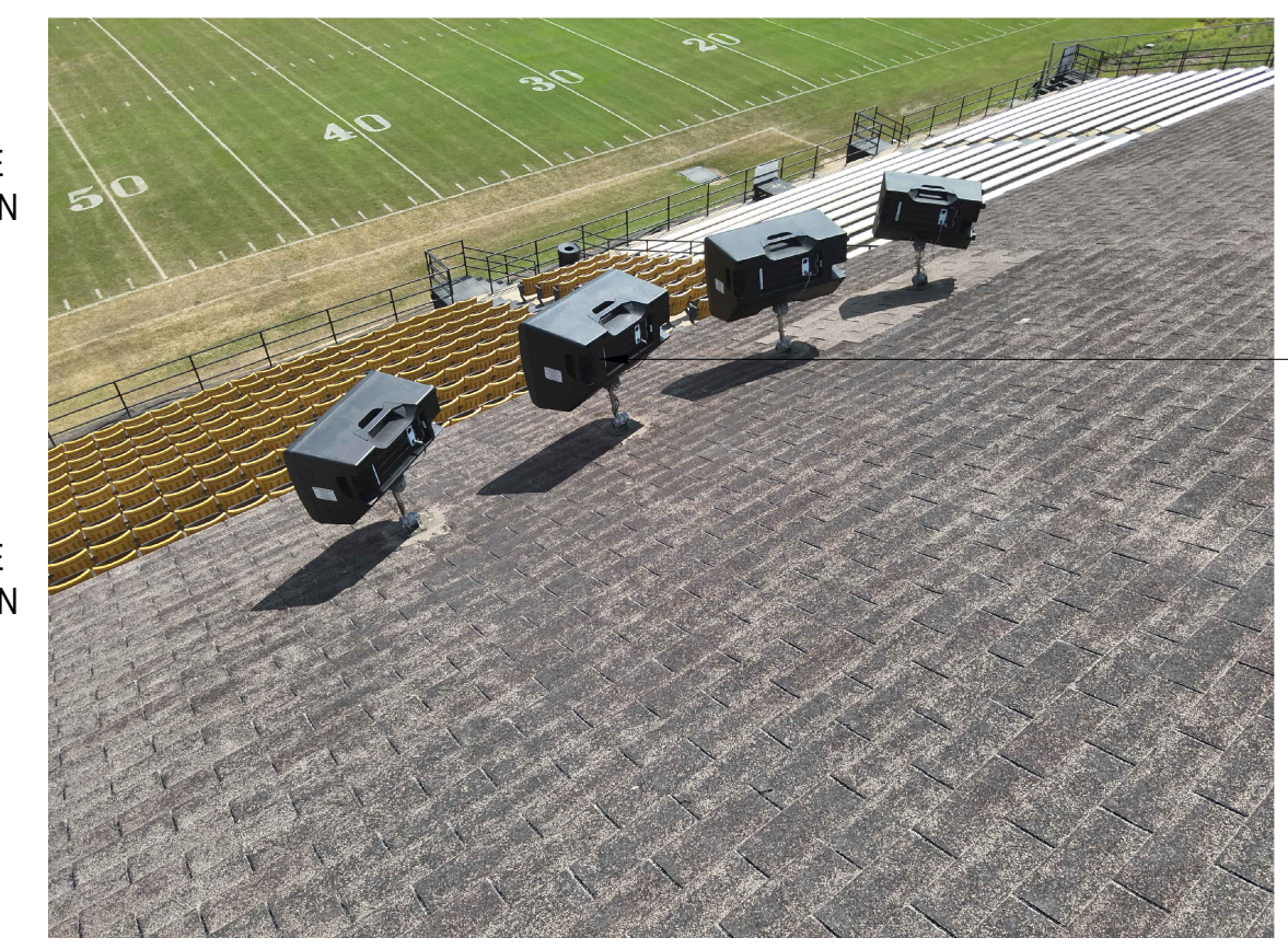
LIGHTS ON PRESS BOX ROOF
